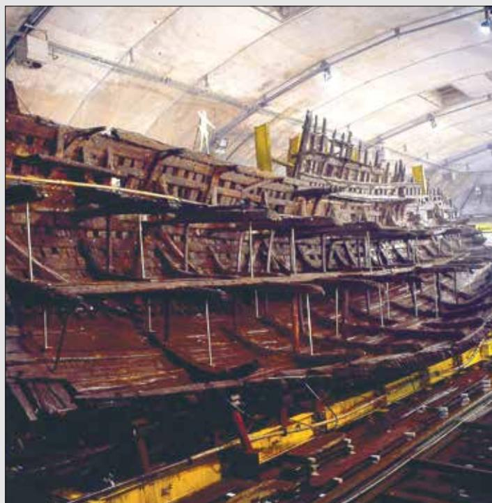
Sprays cover the *Mary Rose* hull with water in 1991. The hull is still on the same yellow cradle that lifted it out of the sea in 1982. It sits on the barge deck, which was cut away when it arrived at the dry dock, and rests on brick piles at a slight angle so that water and PEG solutions could drain away © Mary Rose Trust
