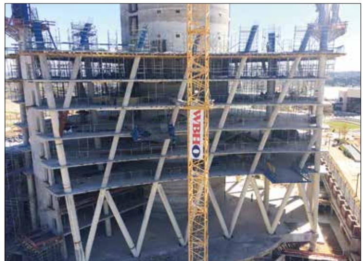
The chosen arrangement of columns under construction, with five across the width of the facade and repetition every five floors. Each column is spiral in shape, but made up of storey-height straight sections with changes of angle at each floor. The counter-sloping columns are purely architectural – to create a V pattern at the lobby level – and carry no loads © Arup
