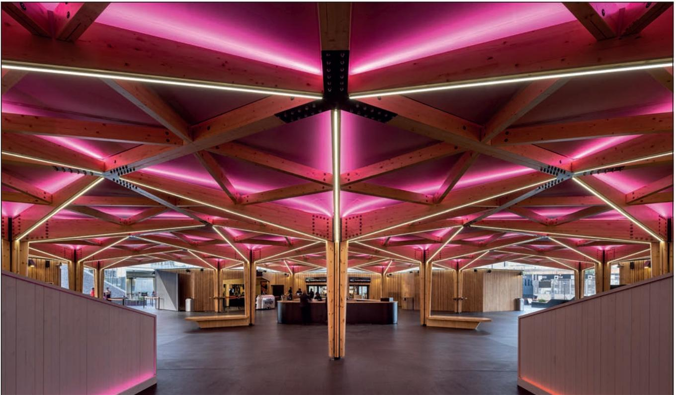
**Timber was the star material of the arena, saving on the building's embodied carbon emissions as no additional finish was needed** © Dirk Lindner, Stufish
