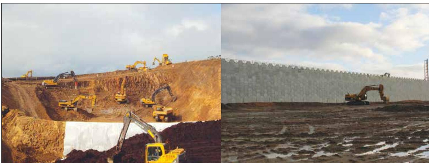
**Before construction could begin on the Shetland Gas Plant, a substantial amount of earth was moved. The soil and peat that was excavated was used to extend the terracing of the bedrock and two large peat stores were designed and created to accommodate the material so that the peat can be recycled to restore the site to its predevelopment condition at the end of the plant's life** © Total
