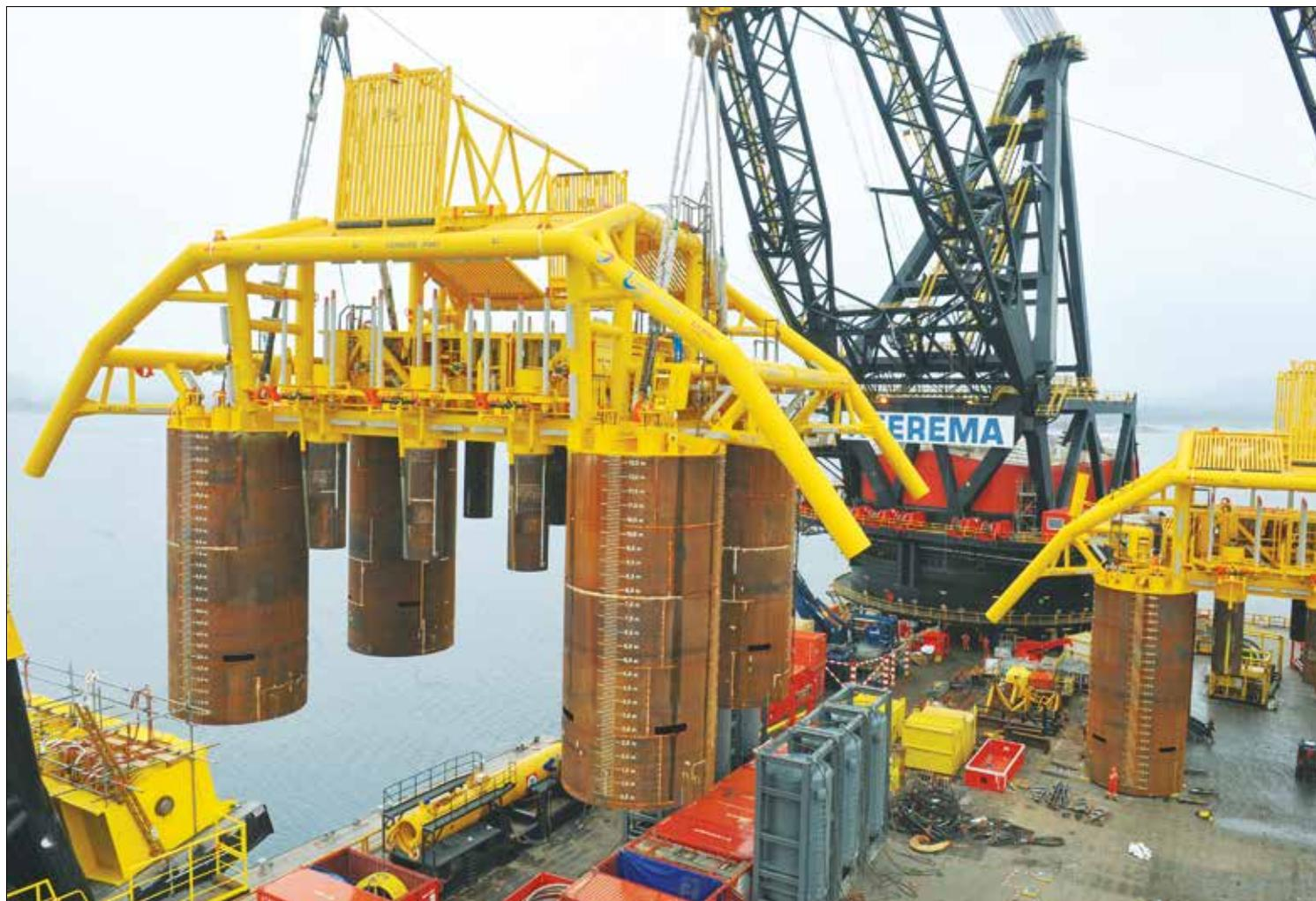
The semi-autonomous subsea production system consists of two six-slot manifold templates that were installed on the seabed on each of the fields. Each manifold is made up of pipes and valves to safely transfer gas from the wellhead into the pipeline © Total
