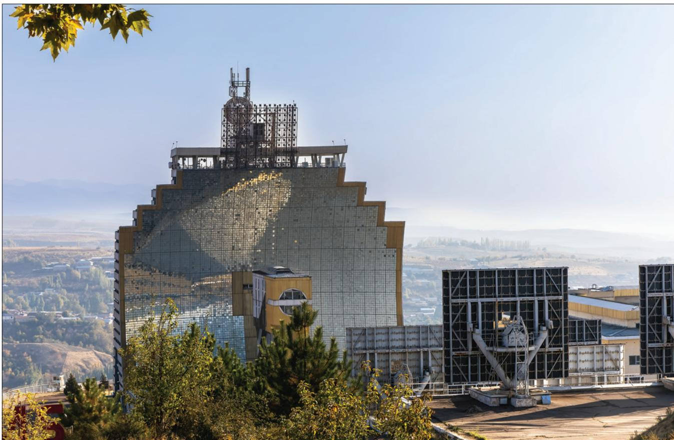
Reaching temperatures of over 3,000°C, the solar furnace at the Sun Institute of Uzbekistan is one way of reaching the high temperatures needed to transform materials. An array of giant mirrors (just seen) reflect sunlight towards the concentrator's 10,700 mirrors, which focus reflected sunlight to a blisteringly hot point. Opened in 1981 during the Soviet era, it was used to make advanced ceramics © Shutterstock
