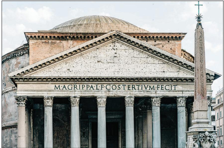
**The nearly 2,000-year-old Pantheon in Rome is made from concrete. The cement they used was typically based on crushed volcanic ash, lime and seawater. Roman concrete is self-healing and has inspired many replacements for Portland cement**
