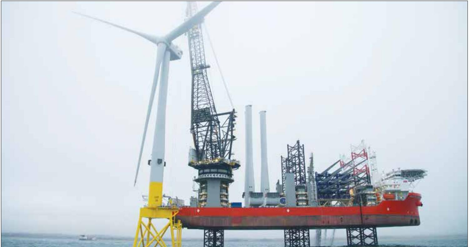
**The Pacific Orca, pictured, is thought to be the world's largest wind farm installation vessel. It transported the turbine from Sweden and installed it in Aberdeen Bay** © TVP Film and Multimedia Ltd
