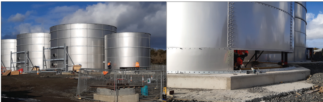
Using steel tanks at the Winchburgh site immediately reduced the project's carbon footprint. The components were prefabricated off site and assembled on site
