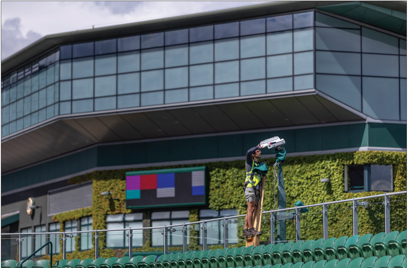
A line-calling camera is installed on No.3 Court. In the background is a Tournament Information Display, which shows schedule, scores, results, and general tournament information for guests. It is the same LED technology as the scoreboards
