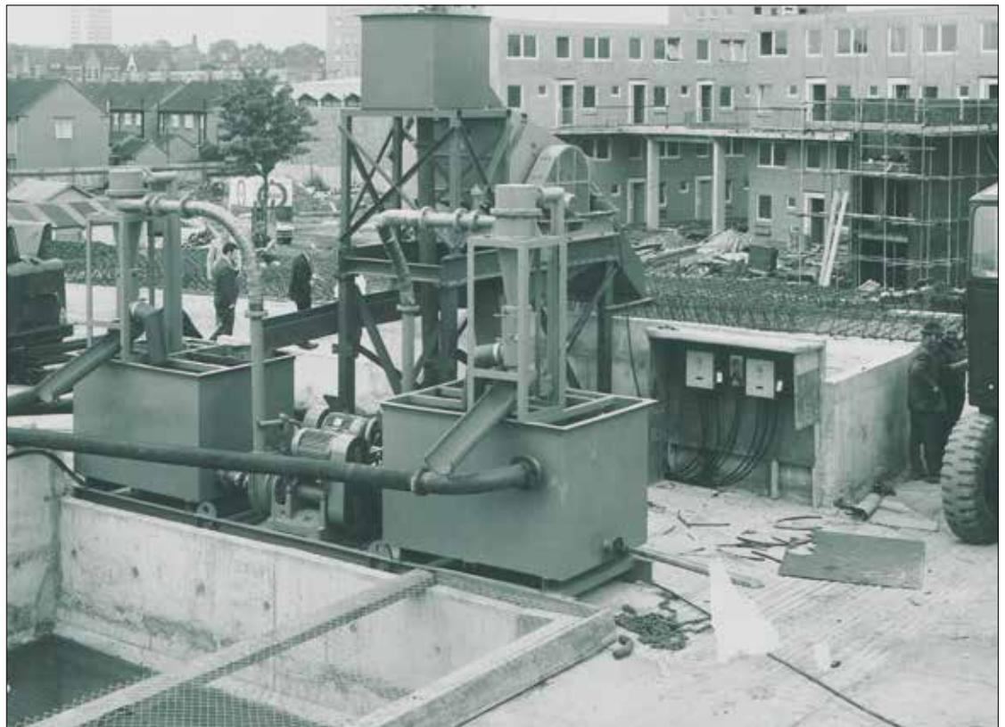
The spoil/slurry treatment plant at the head of the shaft for the New Cross experimental tunnel in 1972, showing twin 12-inch diameter hydrocyclone units and a vibrating screen behind © Institution of Civil Engineers
