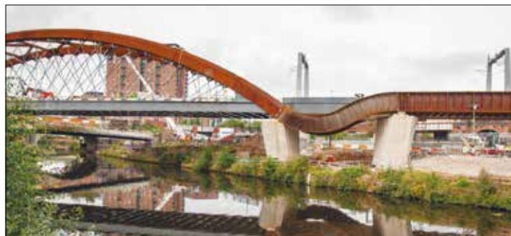
**An integral part of the Great North Rail Project, the Ordsall Chord incorporates the first asymmetric network arch bridge in the world. The Chord uses only 540 metres of entirely new track to connect Manchester's existing railway lines via a brand-new viaduct spanning the River Irwell**
