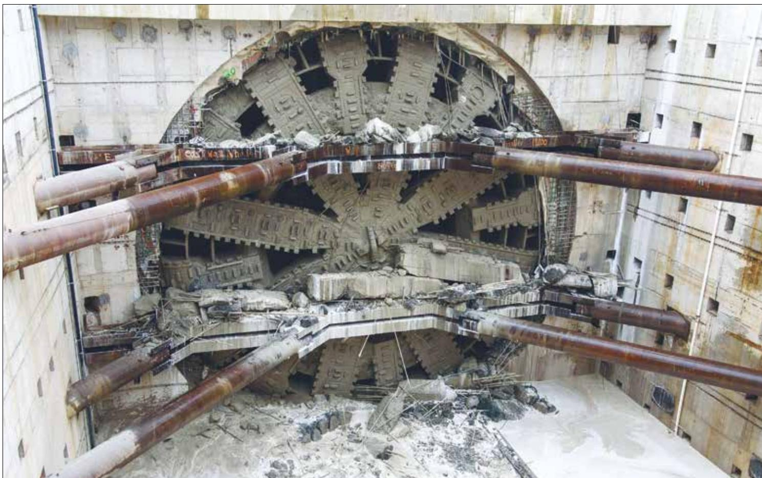
Bertha's breakthrough at the end of the two-mile drive for the Alaskan Way tunnel © Washington State Department of Transportation
