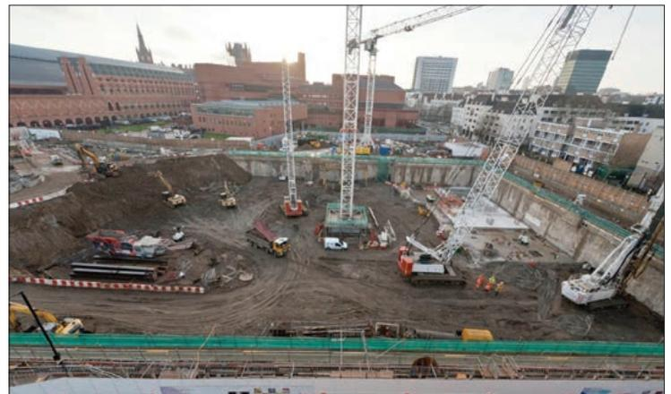
**The basement being excavated down to 8 m depth, 'in the open' to facilitate removal of old Victorian brick and concrete, and with a deep, thick cantilevered concrete retaining wall to protect the sensitive old infrastructure round the sides. At the bottom, a concrete slab was cast and some 260 piles were sunk. Then, construction started on the building above, while simultaneously the remaining two levels of basement were excavated and concreted beneath** © AKT II
