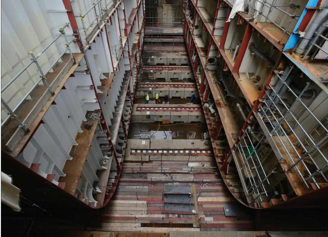
Each of the aircraft carriers have been built in blocks at separate dockyards around the UK before being brought to Rosyth to be pieced together. Massive sections of the aircraft carrier were 'skidded together' with millimetre accuracy. This world record saw 25,000 tonnes of ship moved back more than 17 m © Aircraft Carrier Alliance
