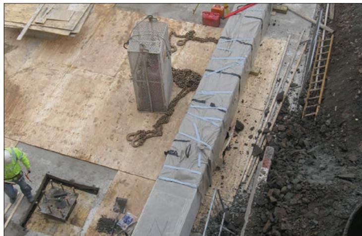
'Top-down' construction for the lower two basement levels, with heavy steel plunge columns supporting the building above while the basement is excavated and concreted beneath. Close to the magnetically-sensitive NMR spectrometers, the steel columns were replaced with precast concrete plunge columns incorporating austenitic stainless steel reinforcement, which reduced magnetic permeability by a factor of around 100 © AKT II
